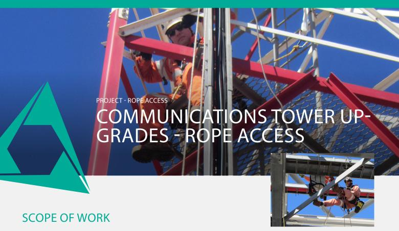
Haztech Solutions where engaged to complete communication tower Electrical Upgrades. The scope of work included Installation of Communication Equipment Cabling and Signalling Systems including testing, hook up and commissioning.
